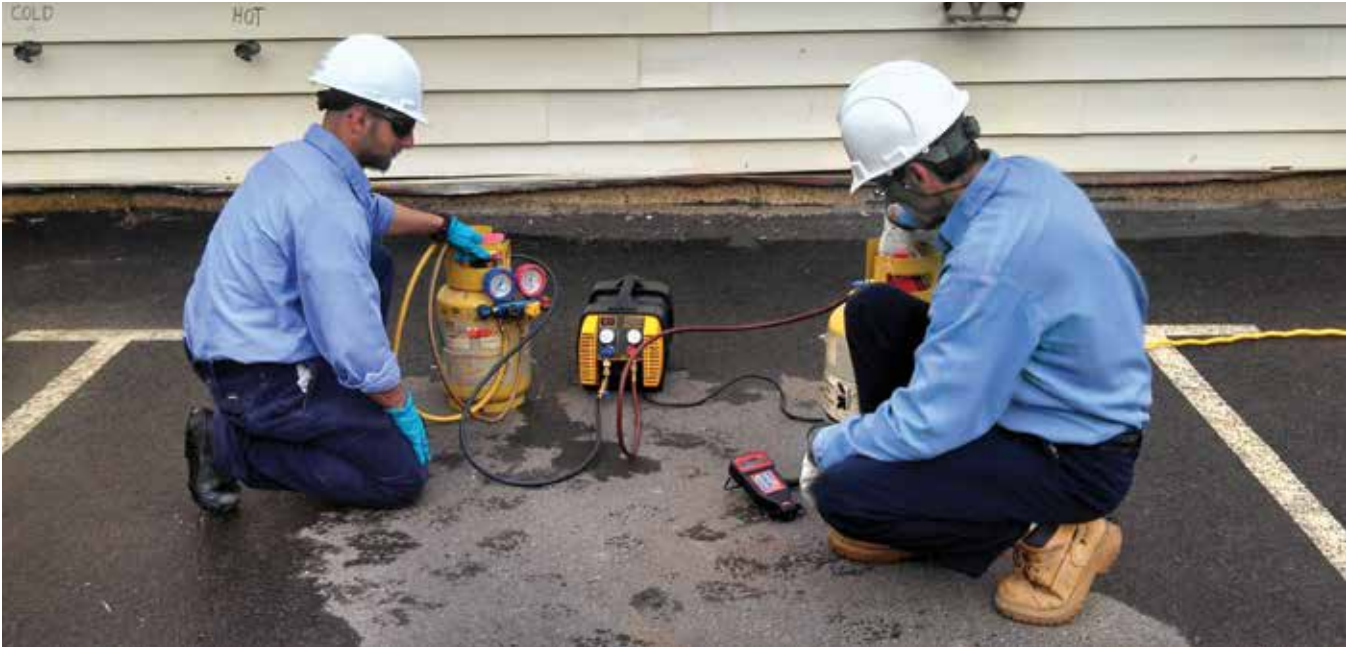
Cpl. Michael Carro (left) trains with HVAC technician Fran Posey at Joint Base McGuire-Dix-Lakehurst, where AbilityOne nonprofit PRIDE Industries provides base operating services. The project currently employs 71 employees with significant disabilities and 28 veterans. Carro was wounded by gunfire while serving in Operation Enduring Freedom. Following his medical discharge, Carro found limited career path options due to his injury. In July 2011, with no prior trades experience, Carro enrolled in PRIDE's trade skills program. The program provides employees with significant disabilities with an accredited progressive curriculum of trade skills development. Eight PRIDE employees with disabilities currently carry certificates or licenses for trades, including plumbing, HVAC, heavy equipment operation and water treatment plant operations.
